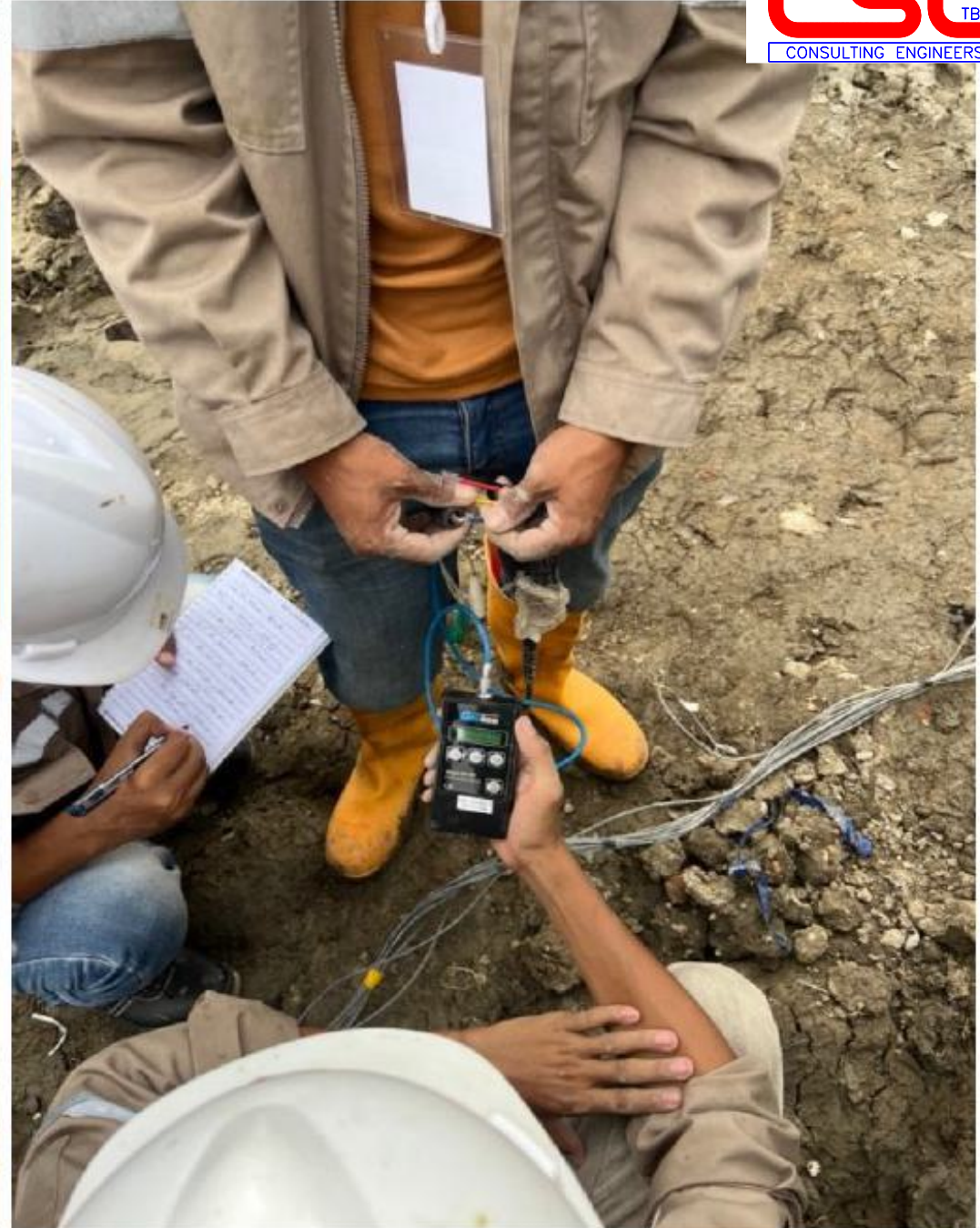
Figure 8: Last Cage & Sensors Checking after Concreting
