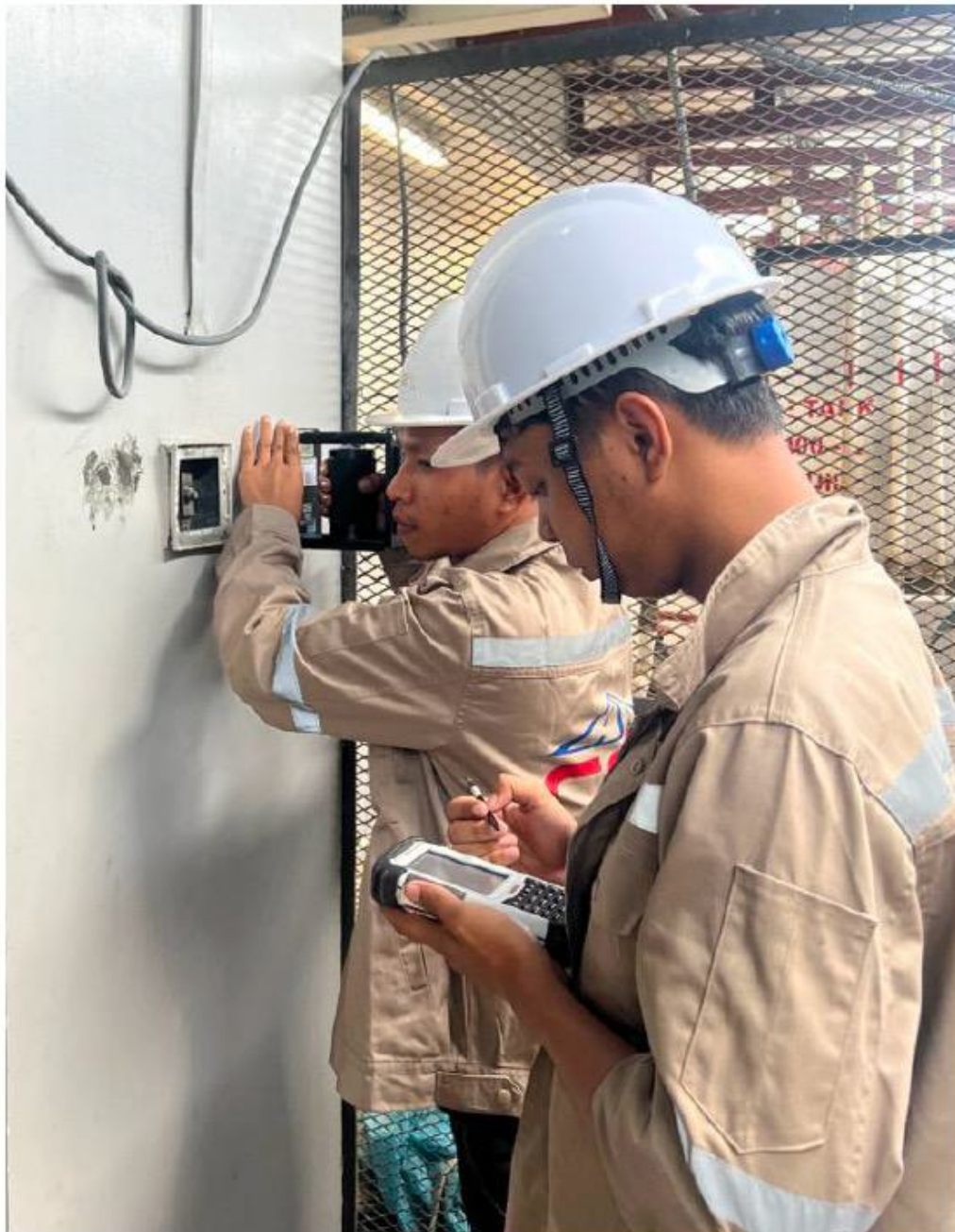
Figure 5: Tiltmeter Monitoring Photos
