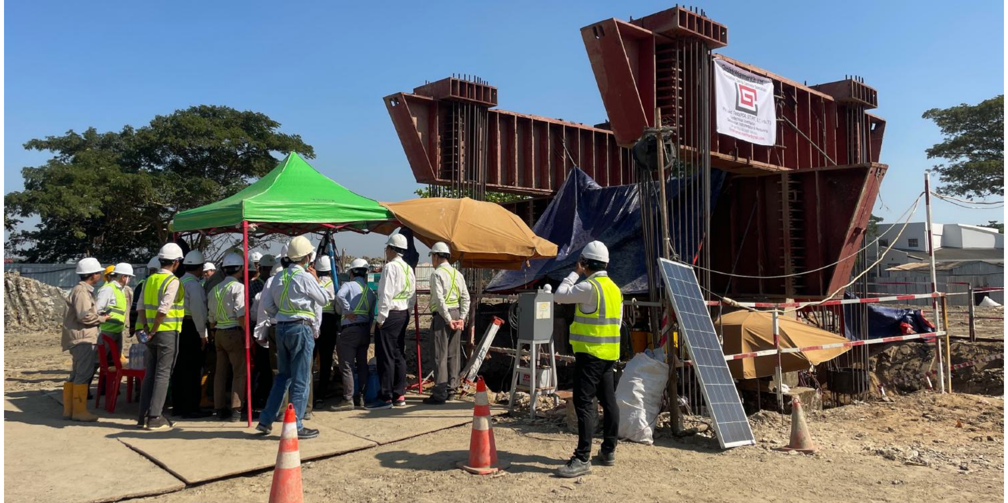
HPBC inspection; Static Pile Load Test for bored pile ASTM D1143
