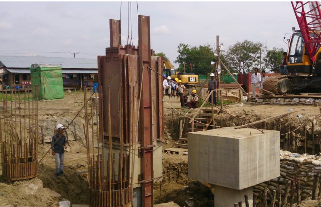
DYNAMIC PILE LOAD TEST FOR PUSHED PILE
