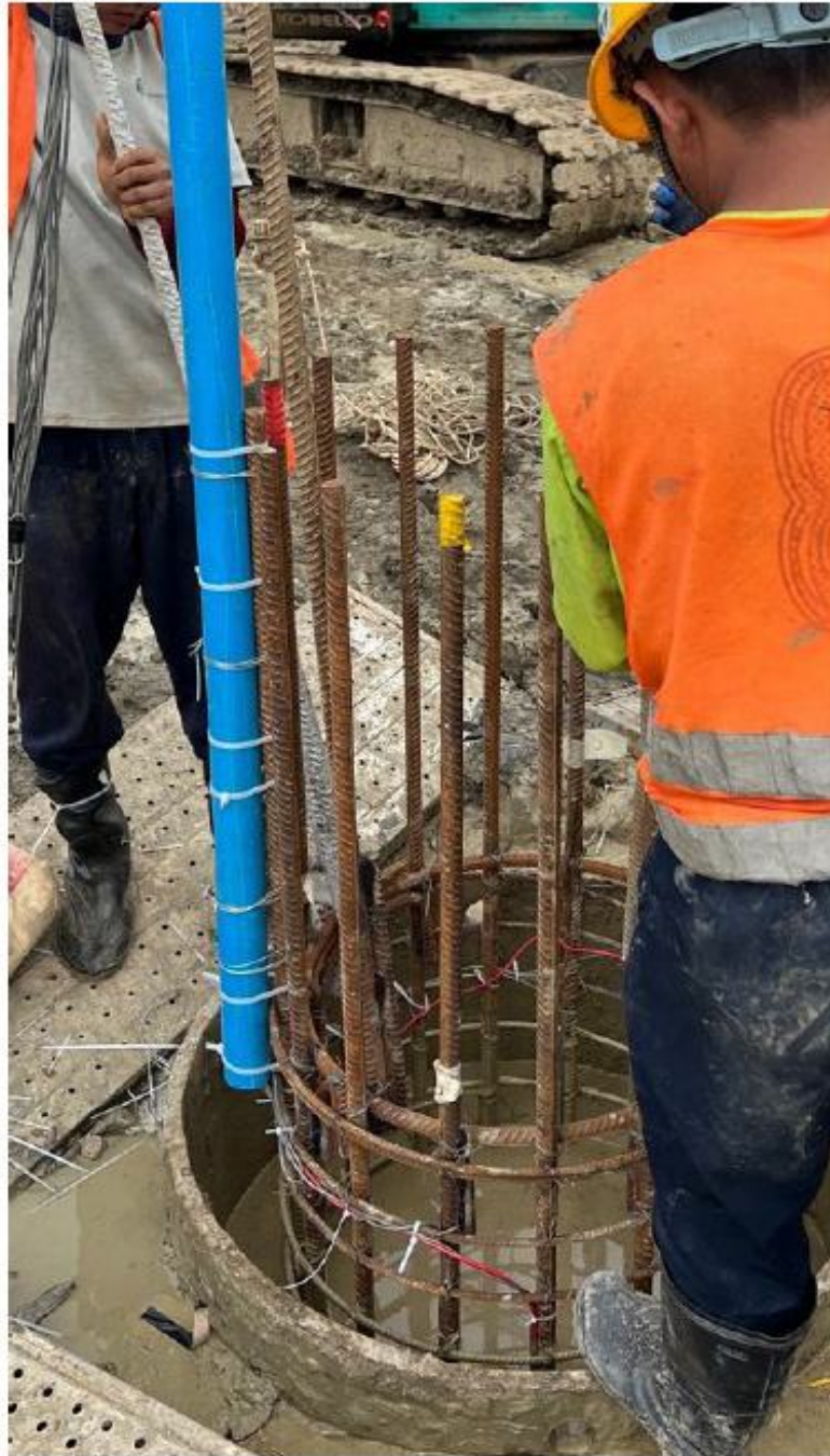
Figure 8: Last Cage & Sensors Checking after Concreting
