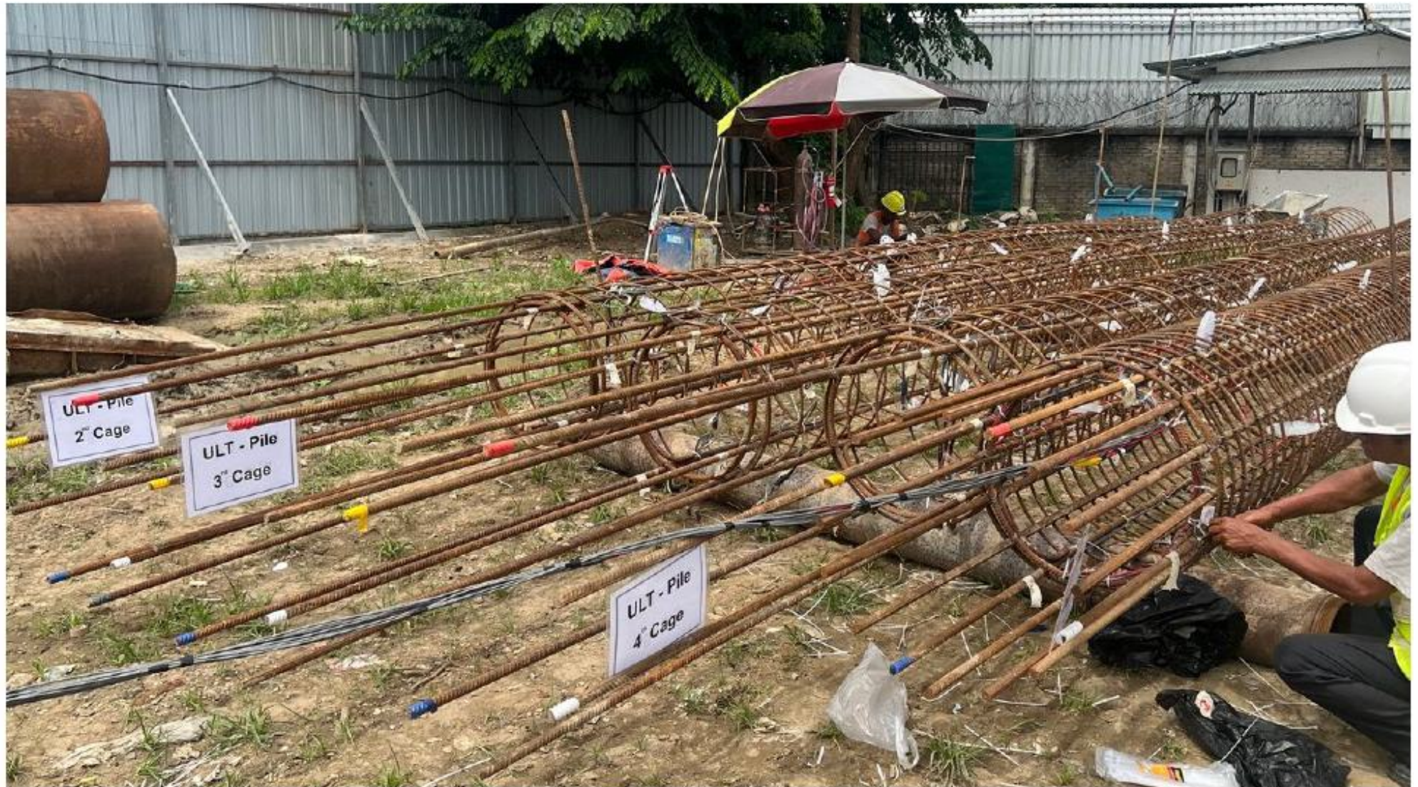
Figure 6: Attaching Cables Rebar Cage
