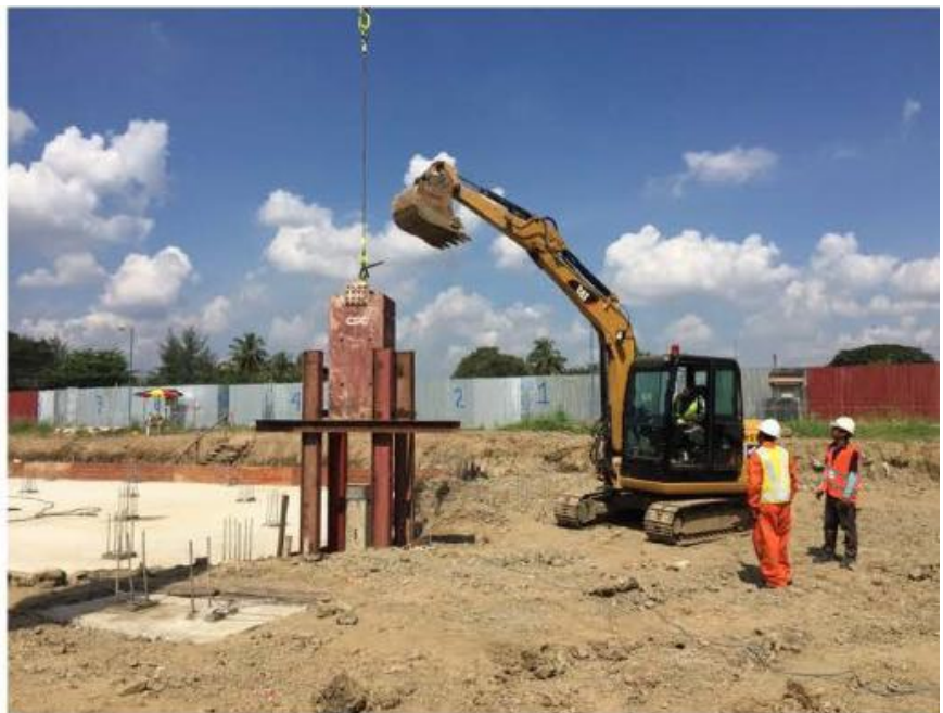
DYNAMIC PILE LOAD TEST FOR PUSHED PILE
