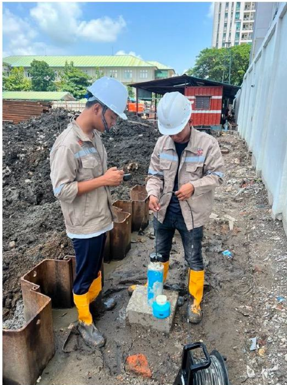
Figure 4: Inclinometer Monitoring Photos
