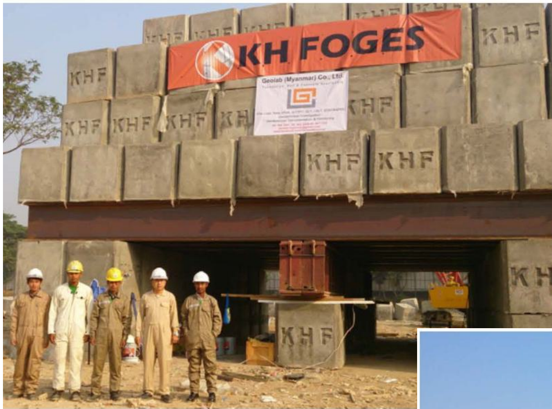
STATIC PILE LOAD TEST WITH KENTLEDGE SYS Shangrila Kandawgyi Project
