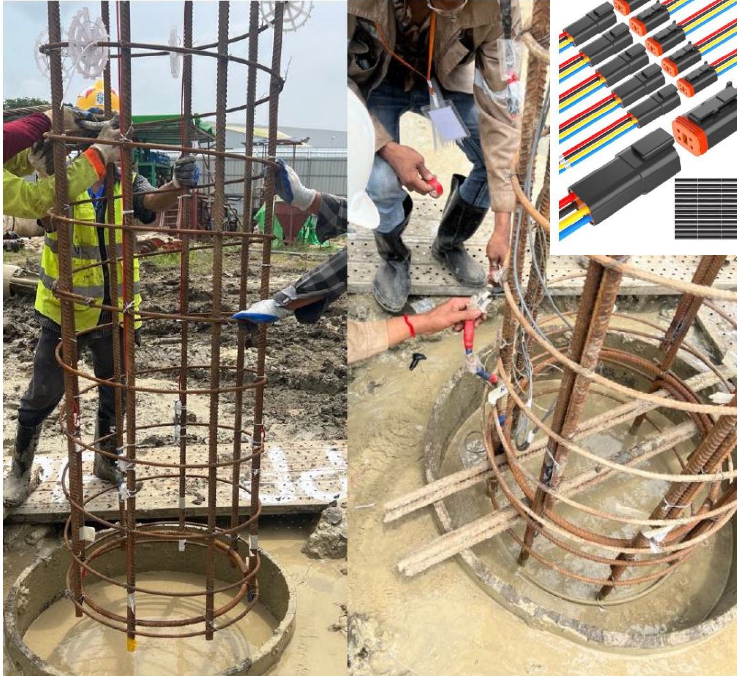
Figure 9: Water Resistant DT Connectors
