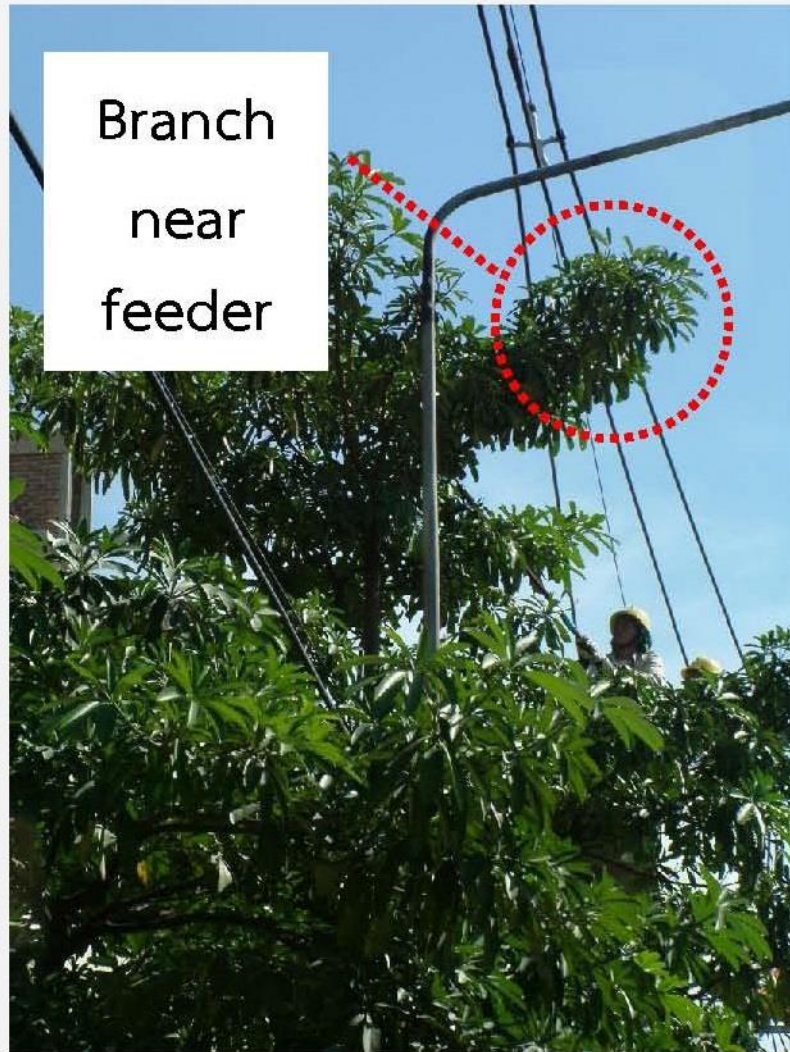
Tree trimming near 24 kV feeder
