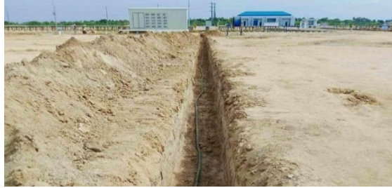
Cable trenches for Cable laying works
