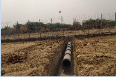
Drainage System Implementation Work
