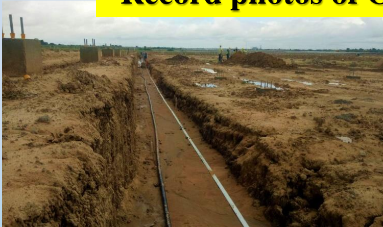
Grounding conductor Installation Work
