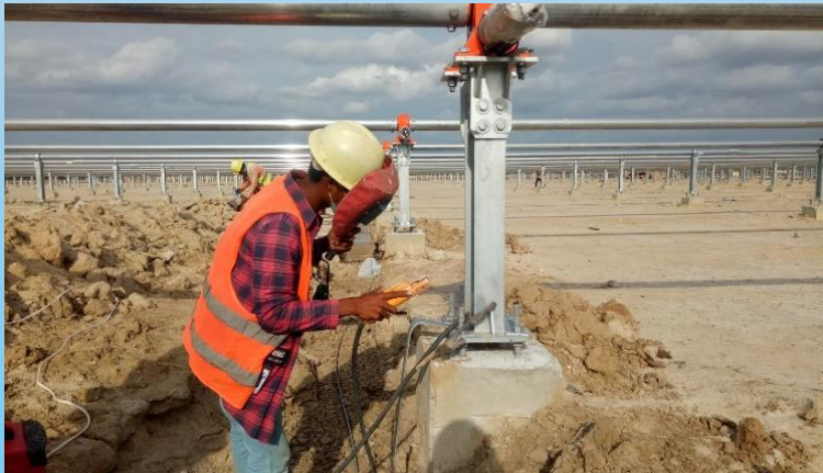
Earthing Connection Installation Work
