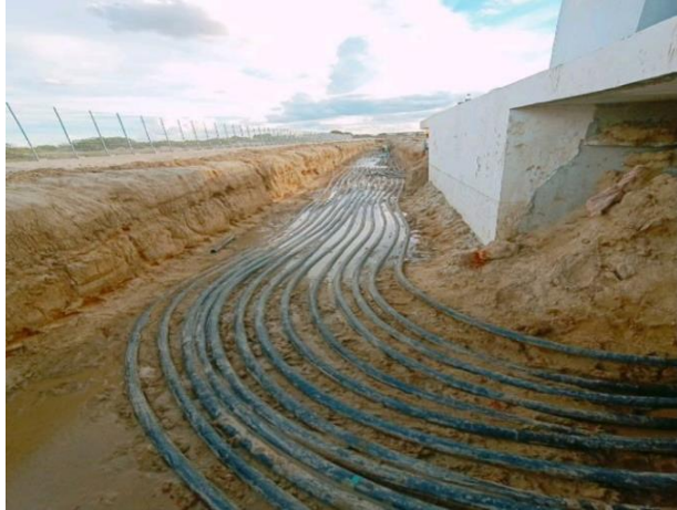
AC cable laying Work
