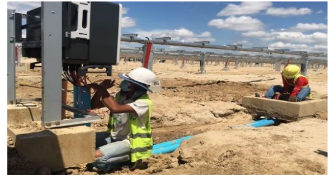
Inverter Side PV Cable Termination Work
