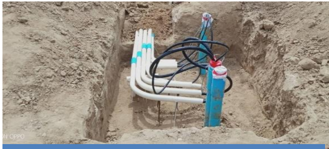
Communication Box Cable installation and Piping Laying Work
