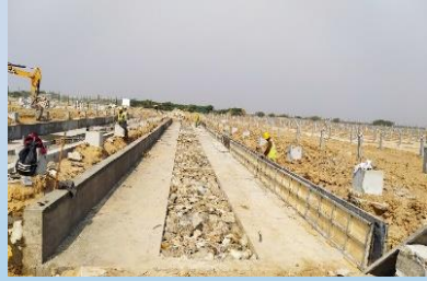
Drainage System Implementation Work
