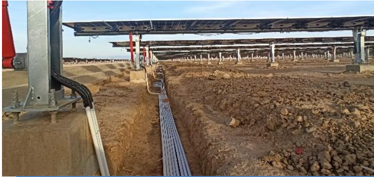
PVC pipe Installation Work for PV Cable Supporting
