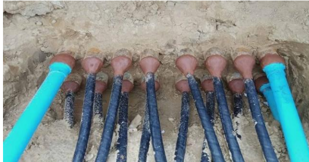
Box transformer underground pipe water proof mud Installation Work
