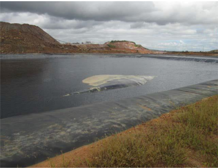
Liner Experiencing an Abnormal Condition
