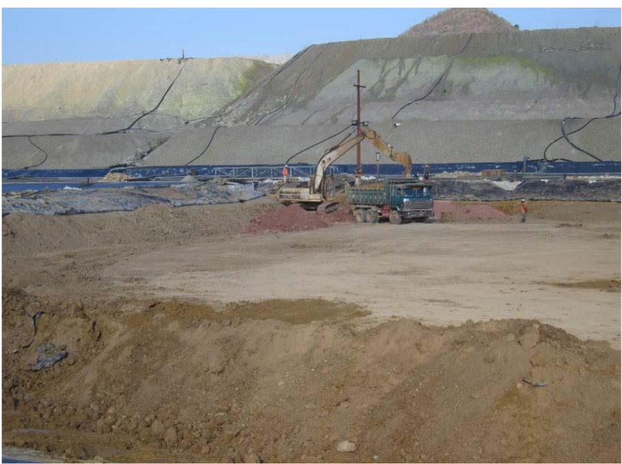
HDPE Pond Repairing
