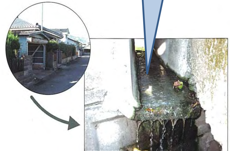
A road gully in tandoku-johkasou installation area in 1970s, (where whitish sludge was attached to)
