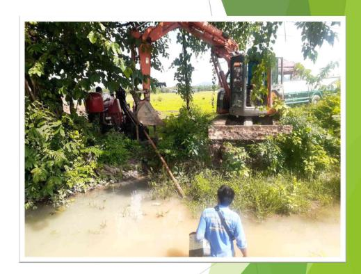
HDD Machine was carried by Crane Truck and Sat @ Work Place
