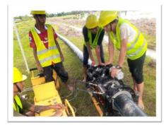
**Grinding both Pipe Ends by Motor Knife**
