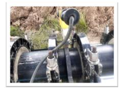
Melting both Pipe Ends by Heat Plate
