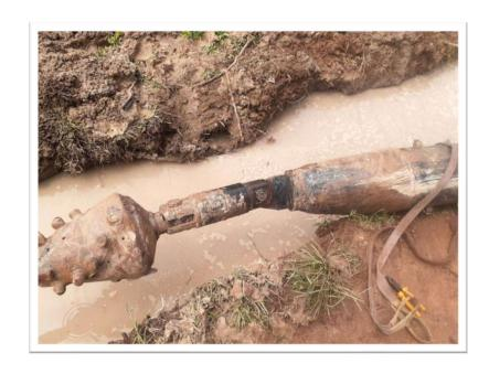
After reaching to End Side, Drilling Bid is changed as Enlarging Bid and Drilling is driven to Back ward.
