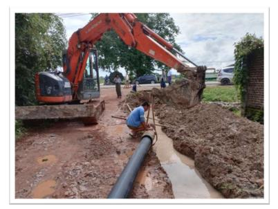
After enlarging the Pipeline-hoe to the Required Size, the pre-jointed HDPE Pipes are connected after Enlarging Bid. And then, the Bid is driven to Back work and the HDPE Pipeline is already pulled through under the Road.
