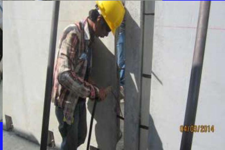
Horizontal Joint Welding
