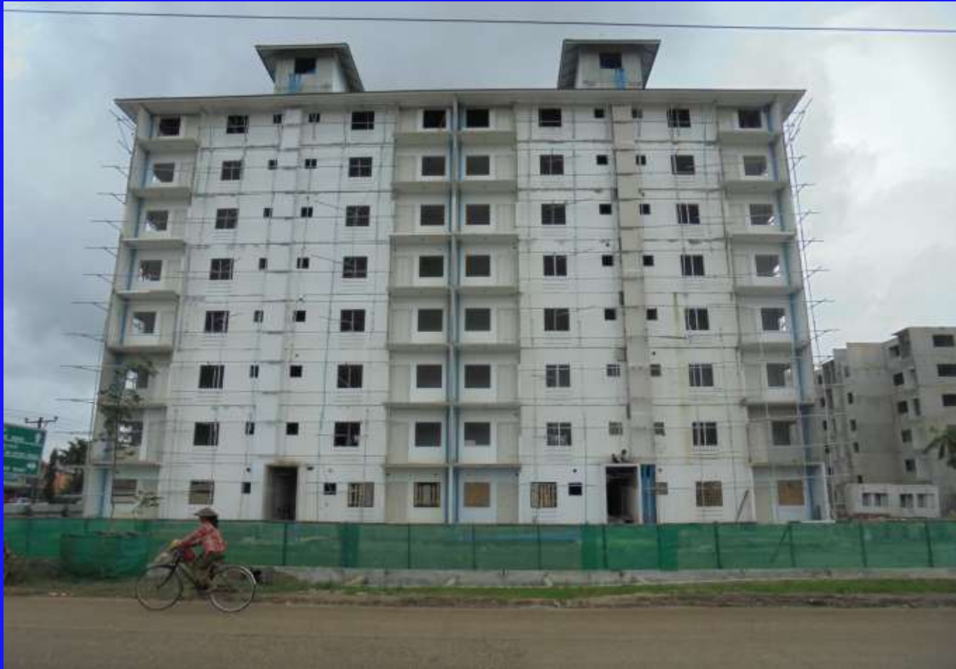
Bldg A1 Back View
