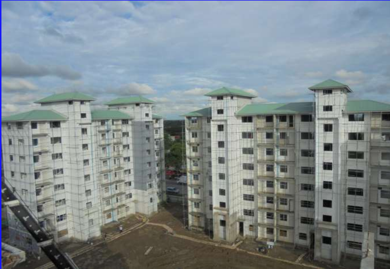
Bldg A1 Front View
