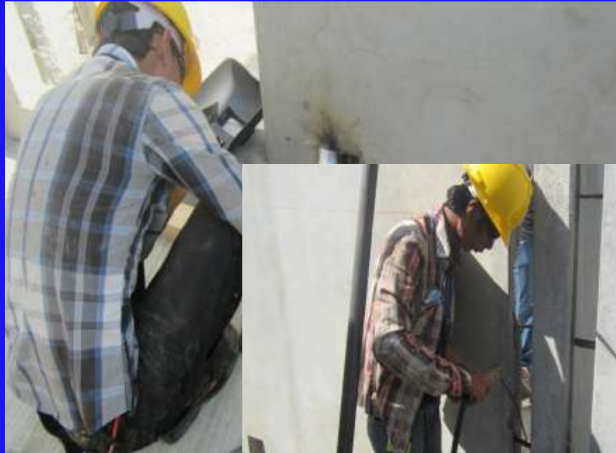
Wall Vertical Joint Welding
