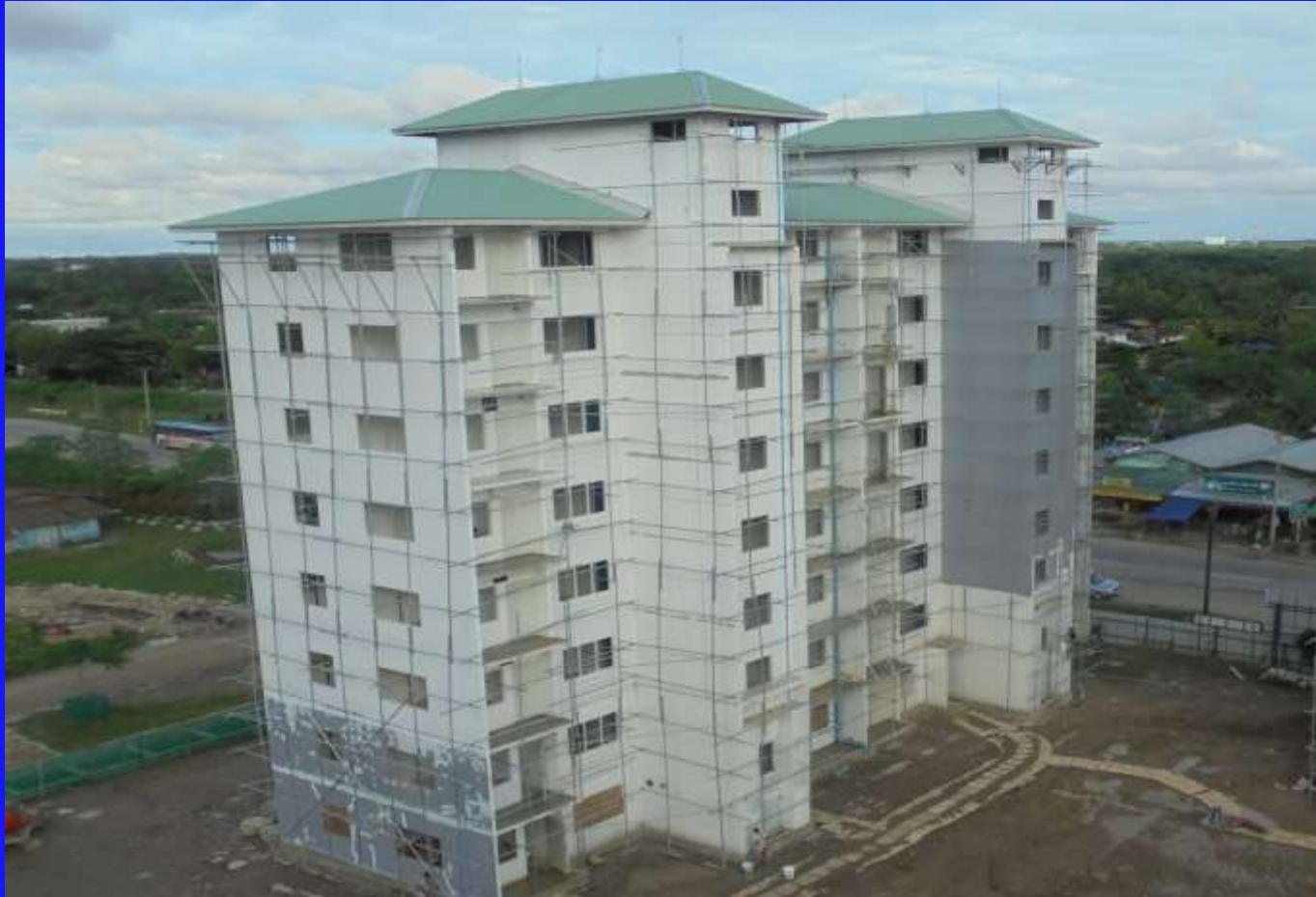
Bldg A1 Front View
