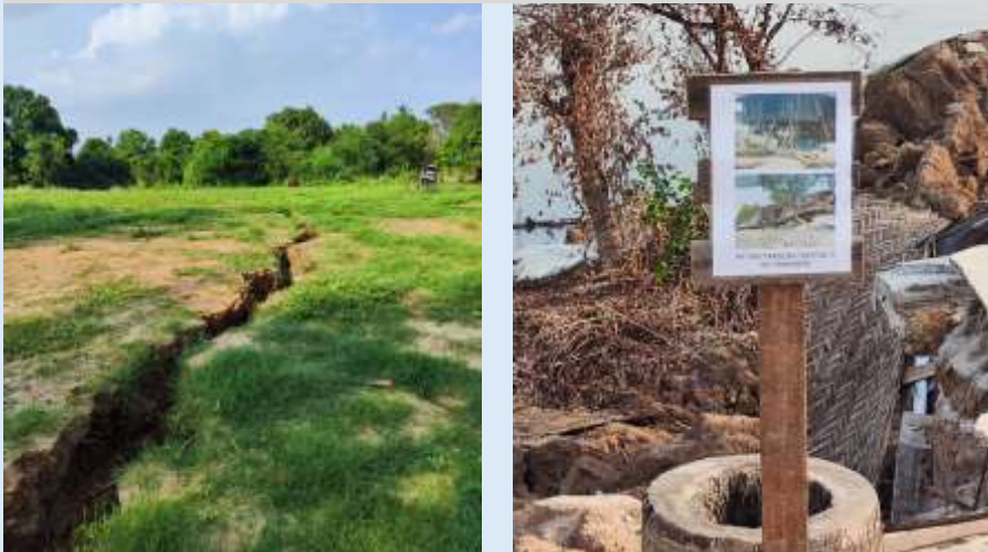
Fault & House Damage in Innwa
