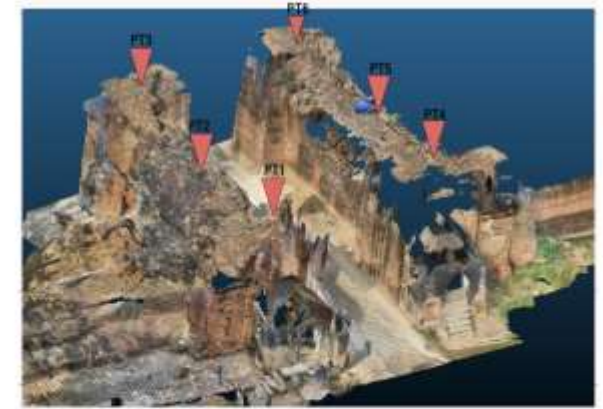
Figure 1: Location of the vibration measurement points from Tharaba Gate
