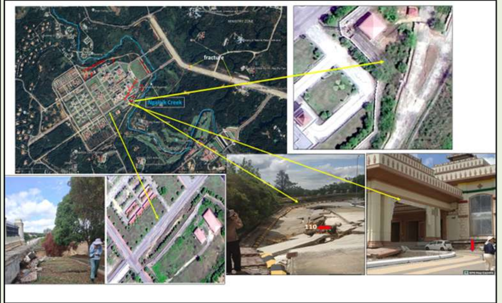
Damages at the Northeast part
