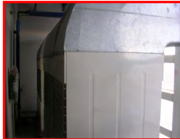
Outdoor units are installed at each story
