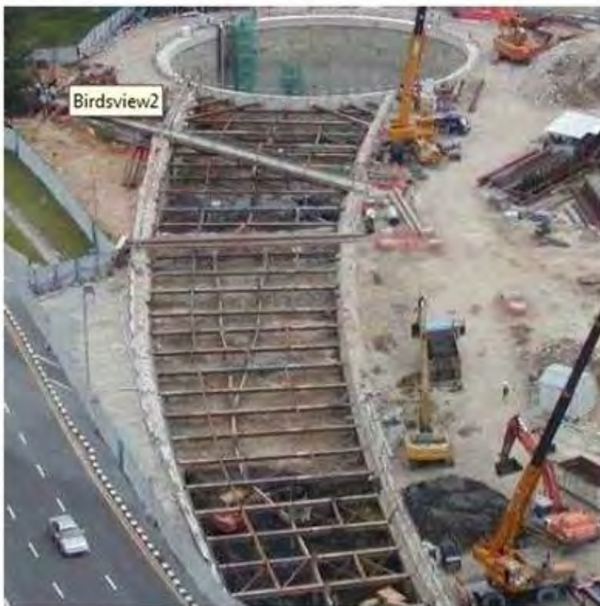
(a). Before collapse
