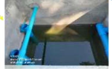
Secondary Sedimentation Tank
