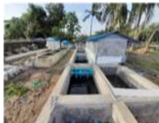
Secondary Sedimentation Tank
