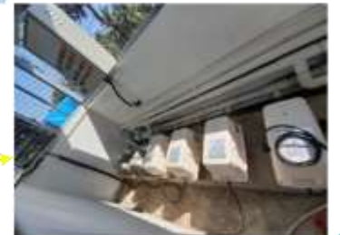
Air Blower House
