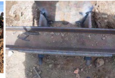
Between soldier pile and waler beam
