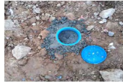
After installation of ground settlement marker
