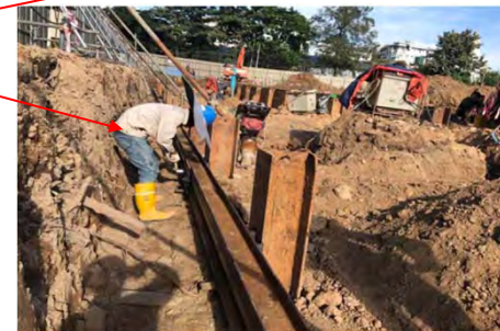
Anchor bar tightening
