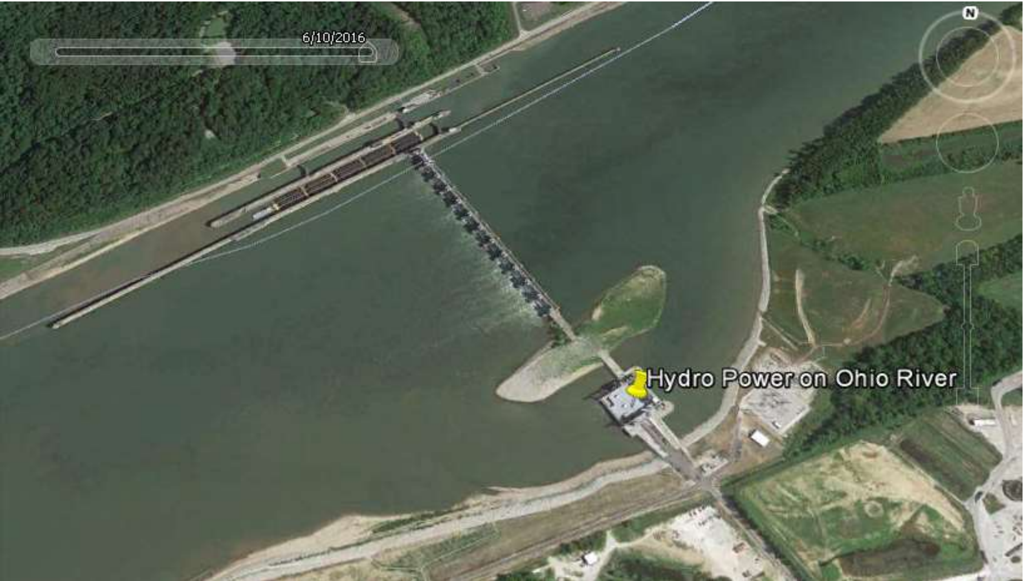
Fig. 8: Ohio River Low Head Hydro, Ship Lock & Turbine House (United States)
