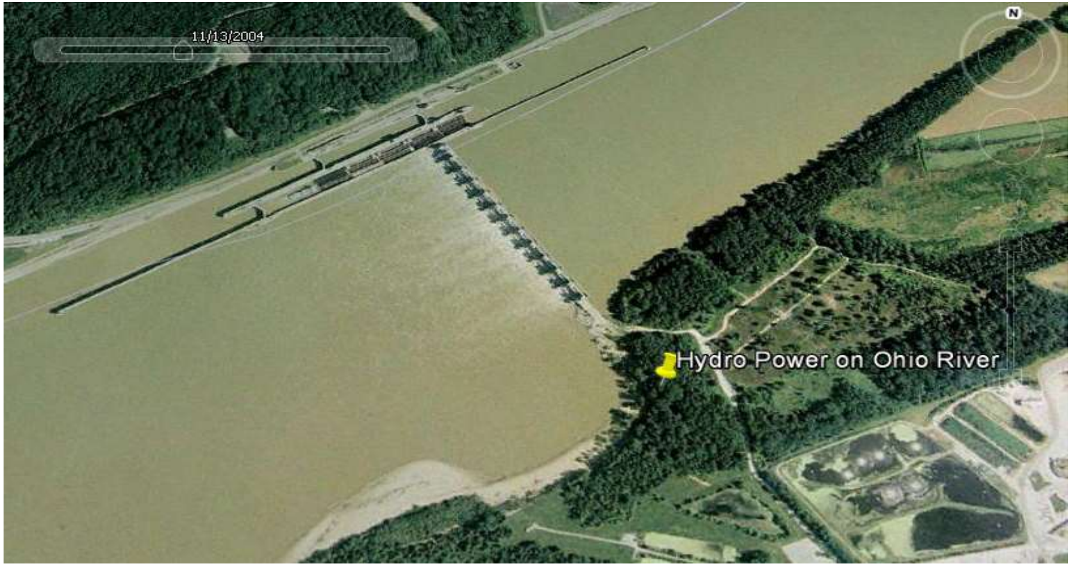
Fig. 9: Ohio River Low Head Hydro, Ship Lock & Turbines. (United States)
