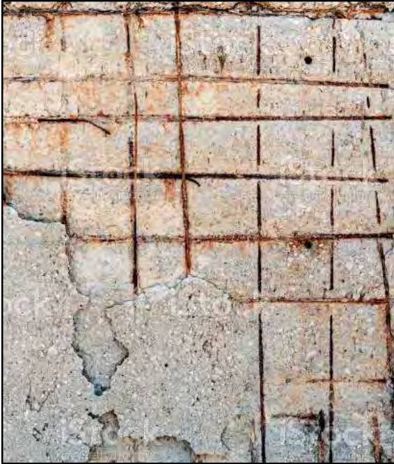
Delamination
