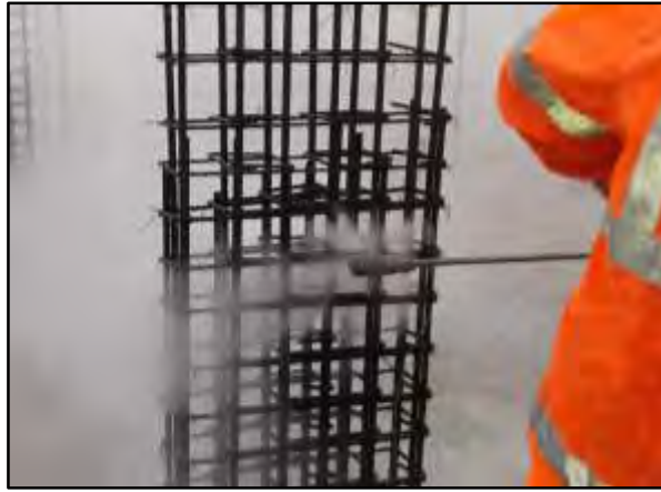
High Pressure Water Cleaning
