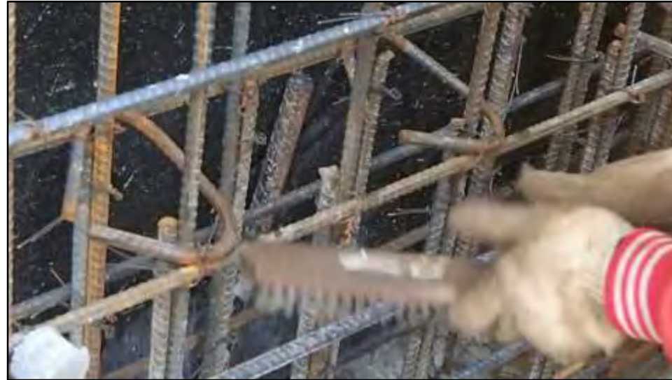
Manual Wire Brushing
