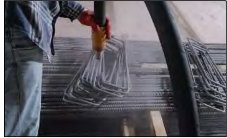
Abrasive (Sand) Blast Cleaning
