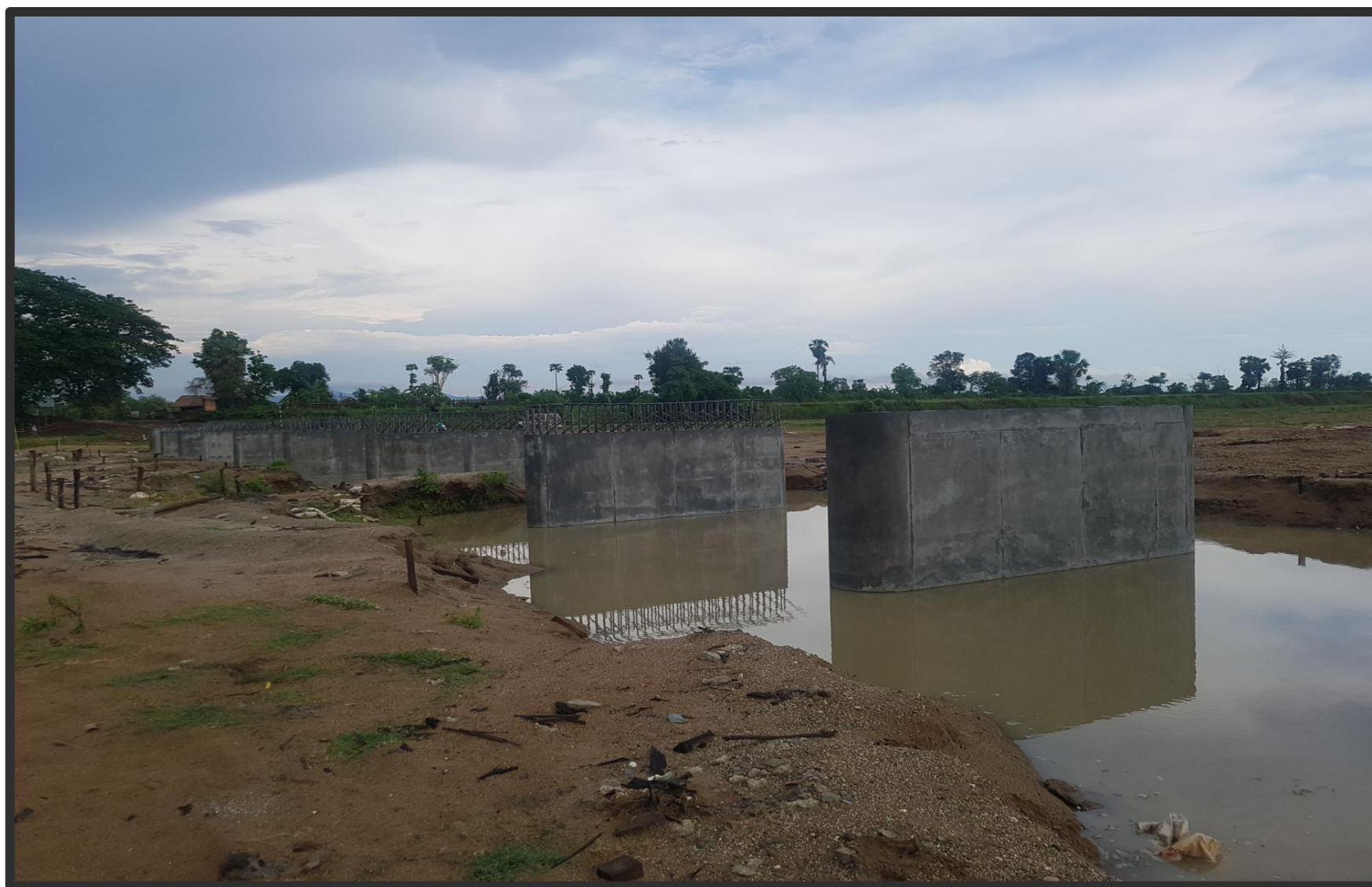
Nant Thar Chaung Bridge
