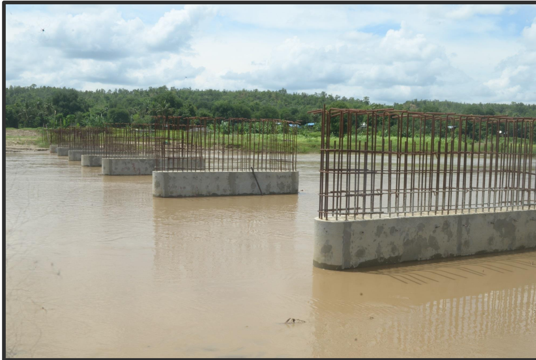
Kyaw Chaung Bridge
