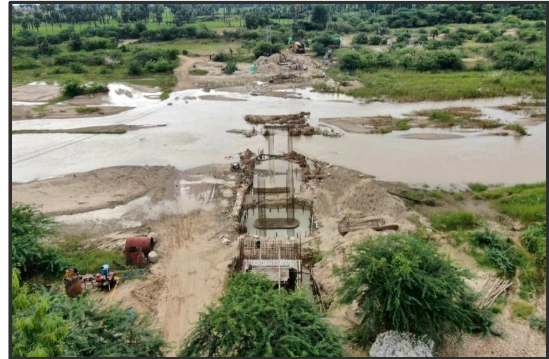
Yamar Chaung Bridge
