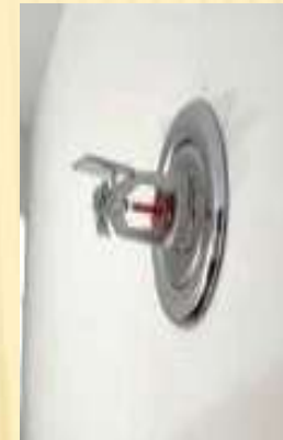
Sidewall Sprinkler
