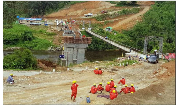
Fig.8 Recorded Photo of Htikha Bridge
