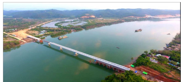
Fig.13 Recorded Photo of Thamote-Lutlut Bridge
