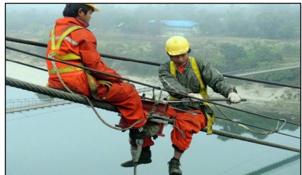
Fig.9 Recorded Photo of Machanbough Bridge
