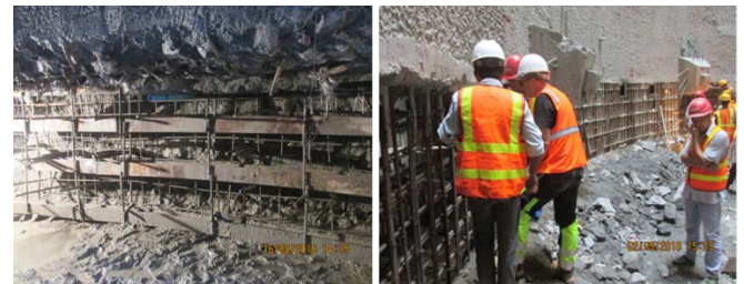
Figure 20 Steel-ribs and primary lining supporting.
