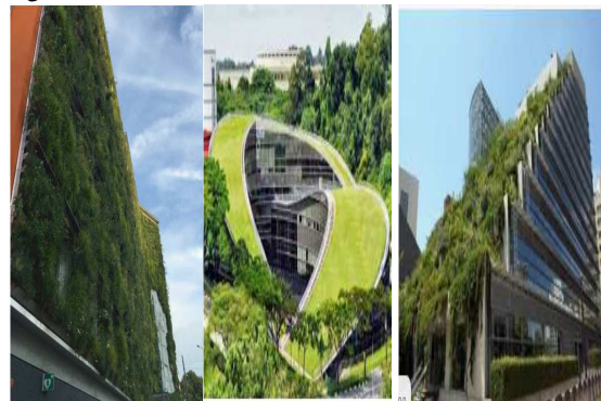
Figure 5. The green wall and green roof
