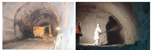
Figure 9 Tunnel excavation and shotcreting
