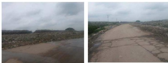
Figure 18: Hard surfaced, well-maintained access road to the disposal site
