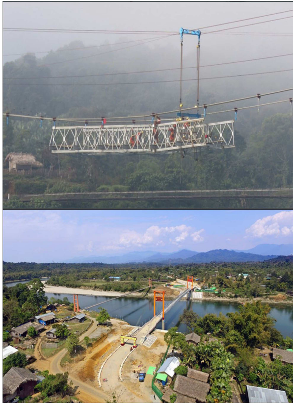
Fig.10 Recorded Photo of Machanbough Bridge
