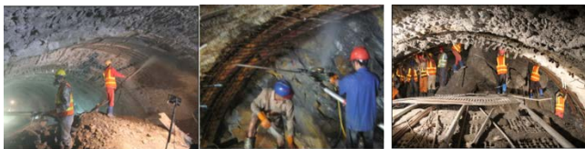
Figure 17 Shotcreting, rockbolting, steel-rib supporting.
