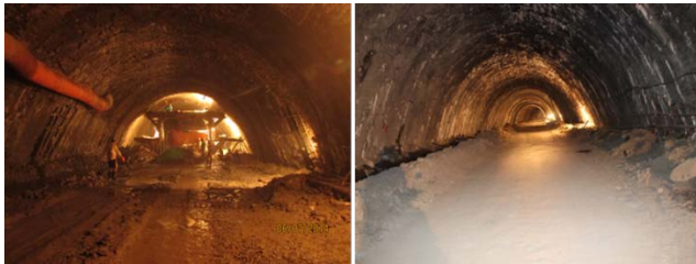
Figure 21 Muddy access and clean access in tunnels.
