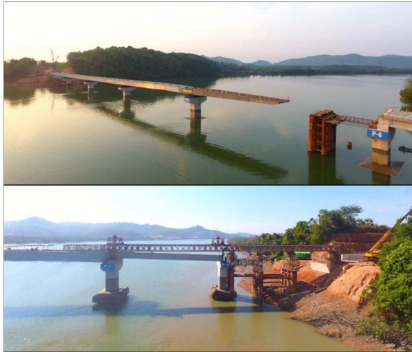
Fig.14 Recorded Photo of Thamote-Lutlut Bridge
