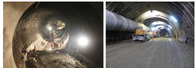
Figure 8 Power supply and ventilation system
