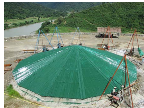
Figure 19 Ring grout for Shaft
